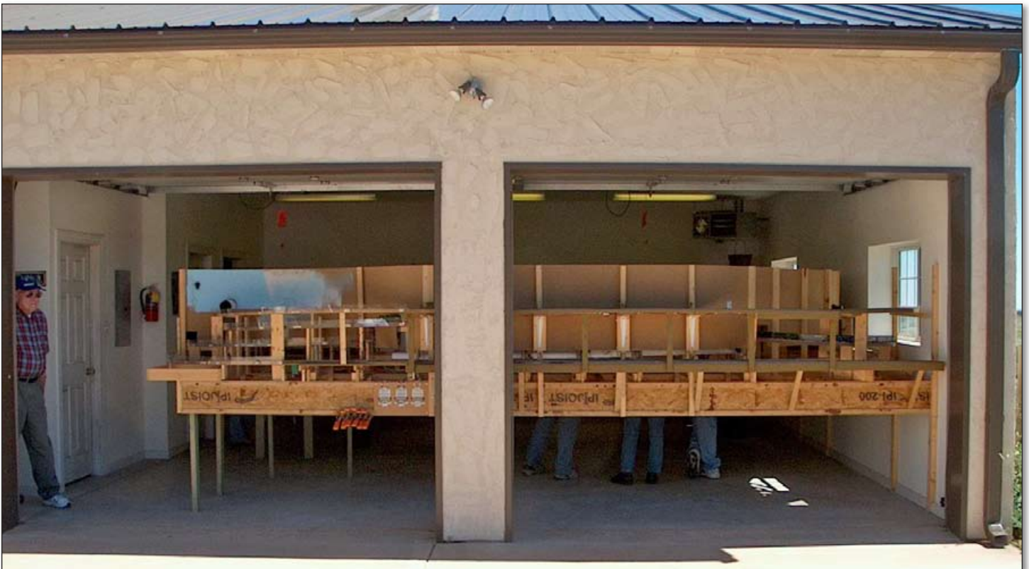
Looking in towards staging yards. Engineered floor joists eliminate all intermediate legs across the width of the layout Dave Zamzow
